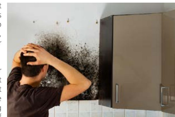
Figure 34: Mold growth
